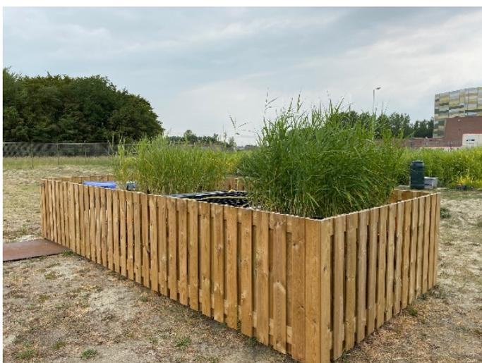
Figure 3: Constructed wetland pilot in Terneuzen, the Netherlands, effectively removing conditioning chemicals from cooling tower wastewater.
