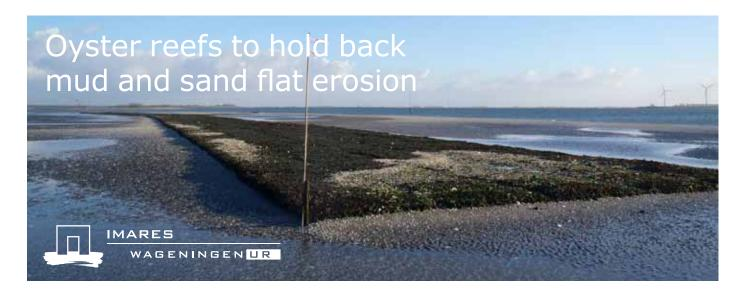
Can oyster reefs hold back the progressive mud and sand flat erosion in the Oosterschelde (Eastern Schedt)? A trial that involved the use of banks of crustaceans to curb wave action and catch silt is being conducted in the Oosterschelde as part of the Building with Nature innovation programme.
