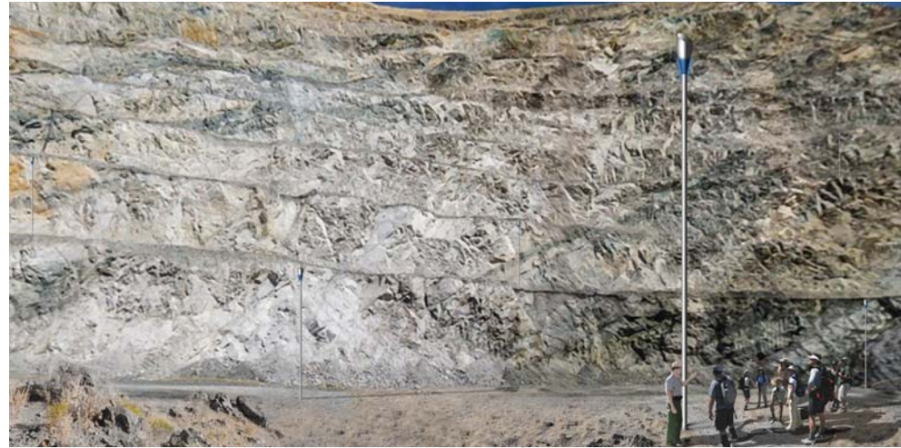
Technological monitoring mast to ensure visitor safety
