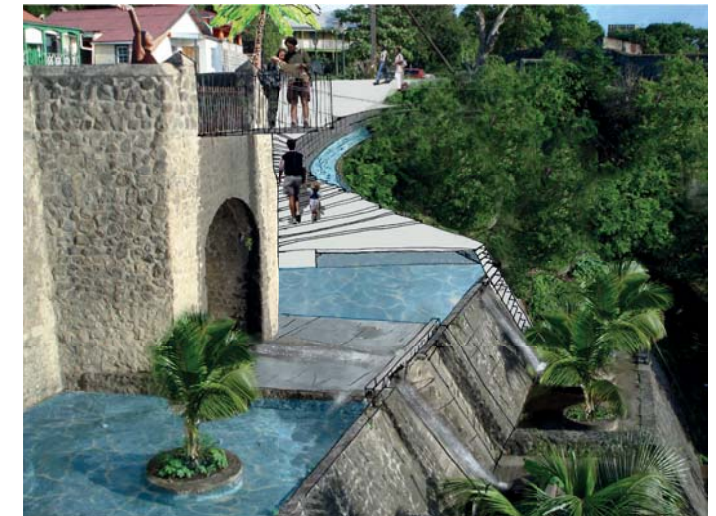
The new stepped plaza improves the connection between Upper and Lower Town and improves the experience
