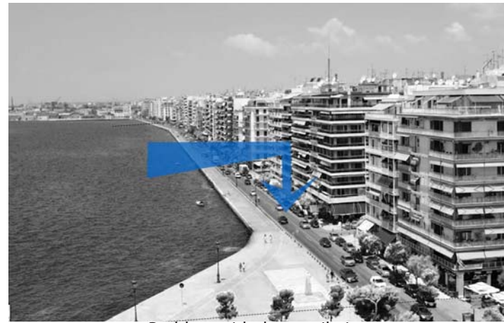
Problem with the ventilation
