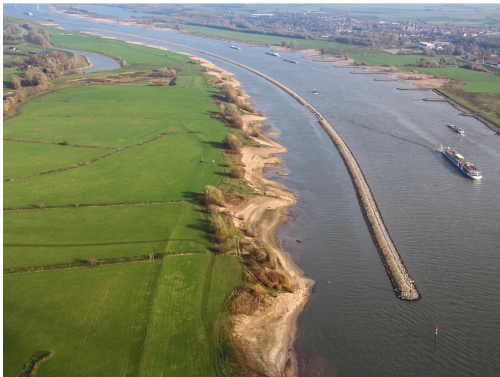
Figure 1: Aerial view on a longitudinal training dam in the River Waal.
