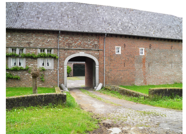
Figure 24: Entrance of Unter Fronrath, one of the oldest remaining carré farms in the area.
