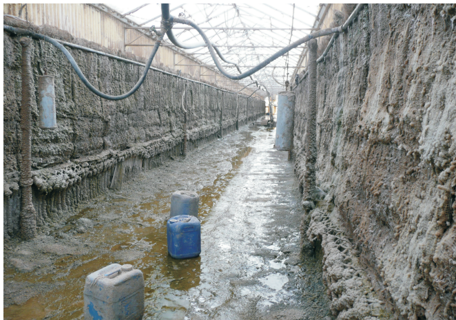
Photo of a pad wall in a greenhouse in Saudi Arabia covered with salt
