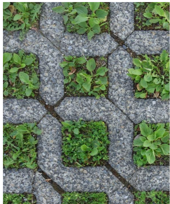
Figure 40 - Permeable bricks can have a hole in the centre, allowing grass to grow.
