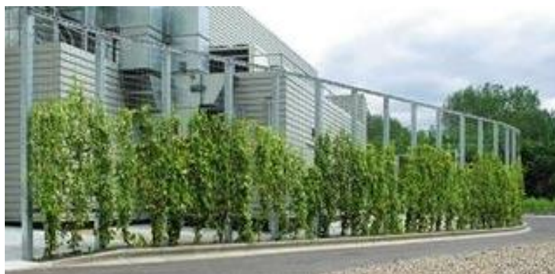
Figure 31 - Example of a free-standing green wall supported by a steel structure.
