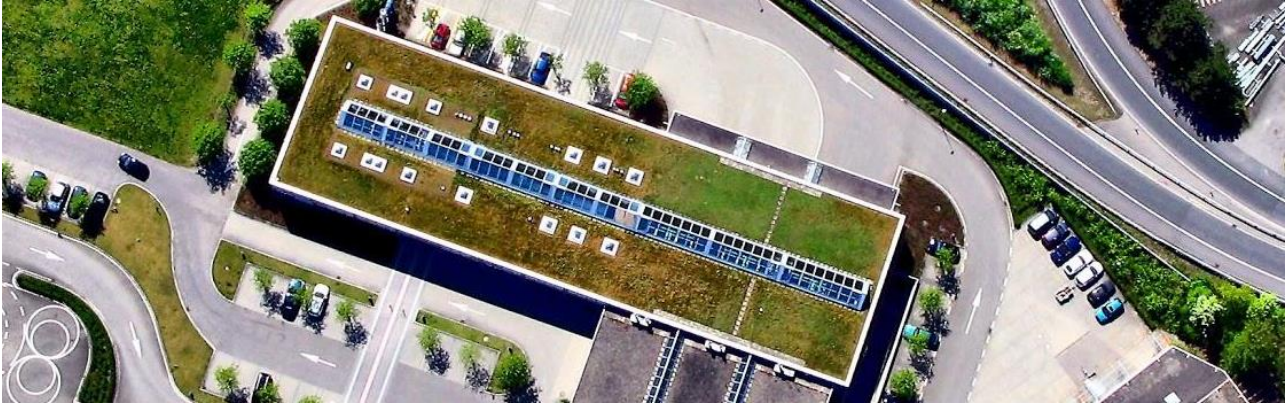
Figure 33 - Example of a green roof with skylights and various vegetations.
