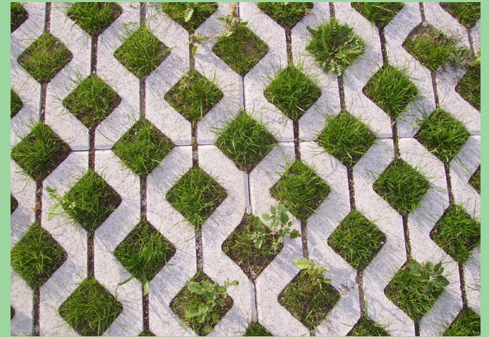
An example of permeable pavement.
