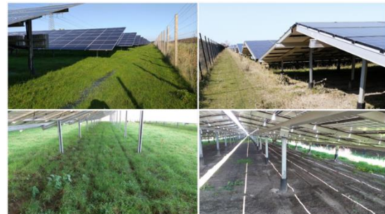
Figure 1: (left) south-facing solar park with ample vegetation below panels and (right) east- and west-facing solar park, with nearly bare soil below the panels. Photo by Alex Schotman via [2].
