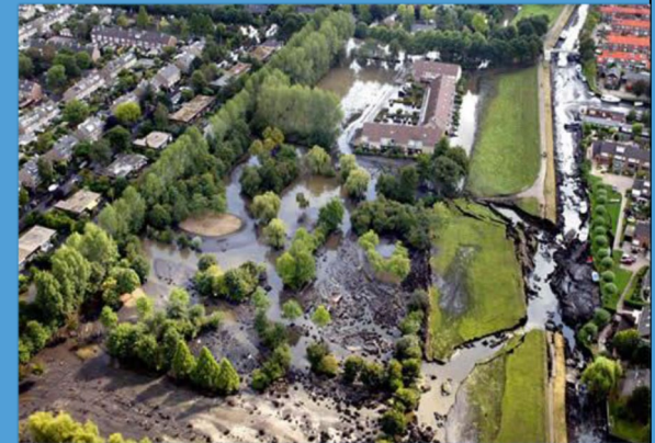
Dike breakthrough Wilnis Netherlands, 2003
