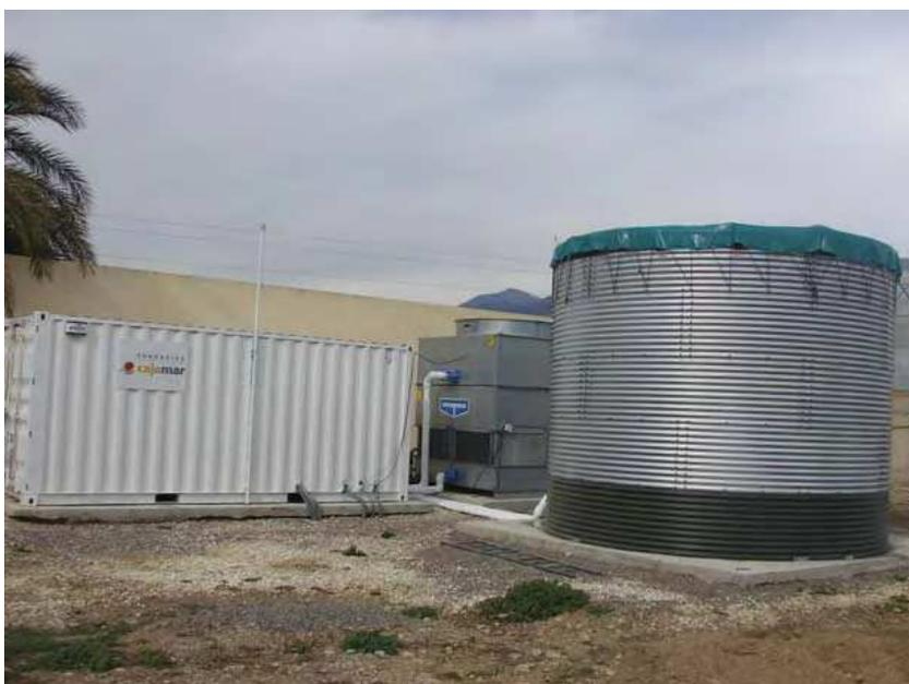
Figure 2.1. Water silo energy store, designed by EEFC to cool and heat a 1000 m<sup>2</sup> greenhouse. The single store is an inexpensive option for the storage of both cold and warm water.
