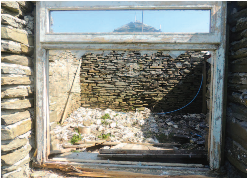
Plate 94. Fulmar corpses litter the floor of the open-roofed enclosure, Cuppin, Papa Westray, Orkney, May 2016; note the window was previously intact. © Tim Dodman
