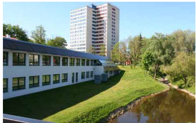
Main building and Student hostel.
