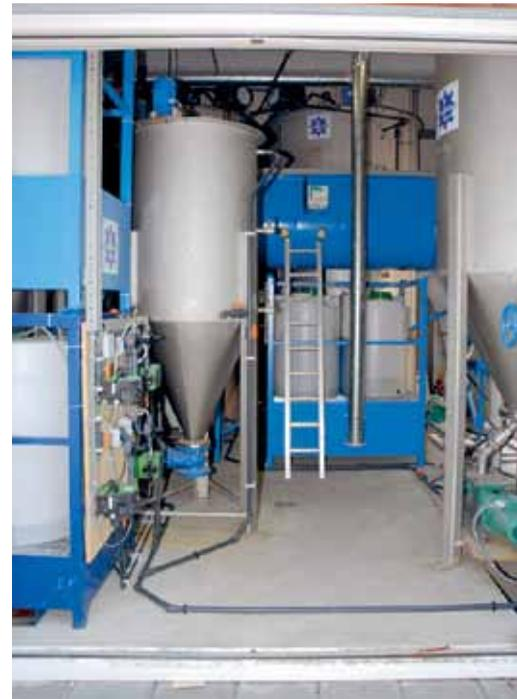
The UASB reactor for the treatment of black water from 32 households is placed in a garage. Photo: Brendo Meulman.
