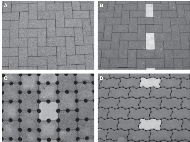
**Fig. 1** Concrete pavings used in this study: paver type and corresponding laying pattern (in brackets). (A) Conventional pavers (herringbone pattern), (B) porous pavers (herringbone pattern), (C) pavers with draining holes (running bond) and (D) pavers with enlarged joints (running bond).
