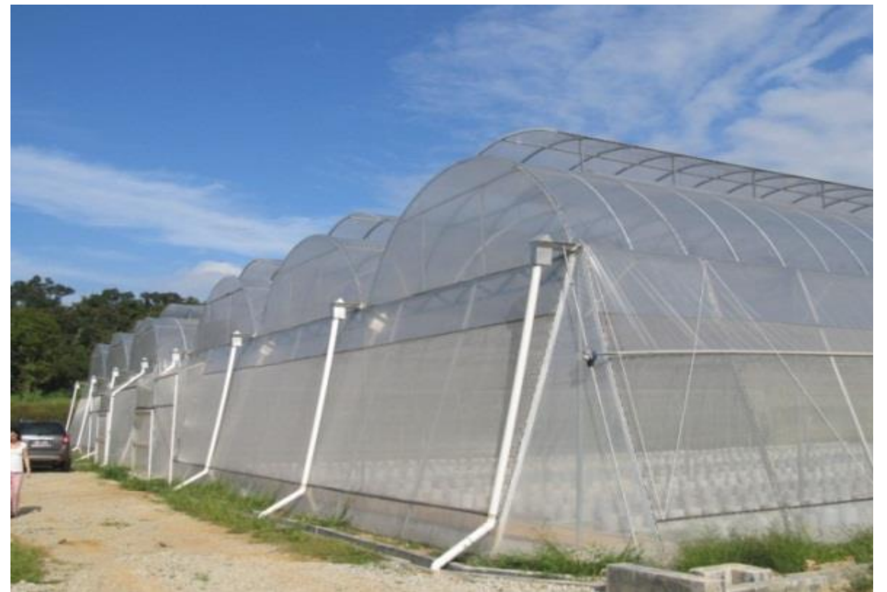
A local constructed greenhouse for lowland tropics (Malaysia)
