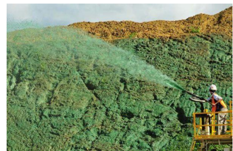
Figure 4: Hydroseeding in Indonesia Source: GPFLR, 2013
