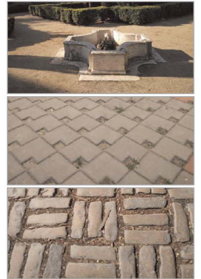
Figure 14a, 14b and 14c: Porous, open cell, and interlocking pavements (From: Silva, 2019)
