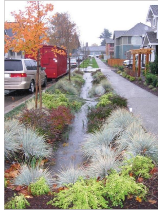
Figure 13: Bioswale transporting runoff after a rainstorm in Michigan, USA (Watershed council, 2019)
