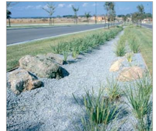
Figure 15: Infiltration trench between two roads in Georgia, USA (Georgia planning, n.d.)
