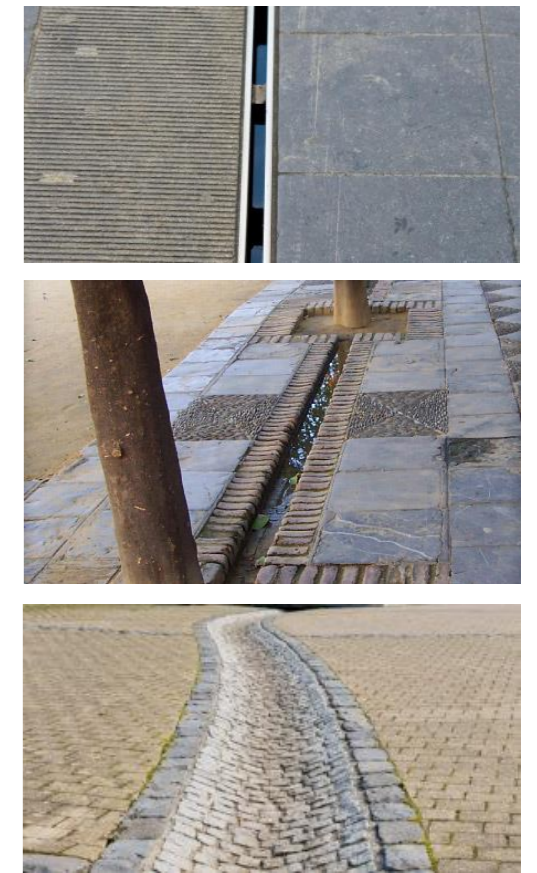
Figure 17a, 17b and 17c: Differently shaped open street drainage channels (City & County of San Francisco, 2015; Atelier GroenBlauw, 2020)
