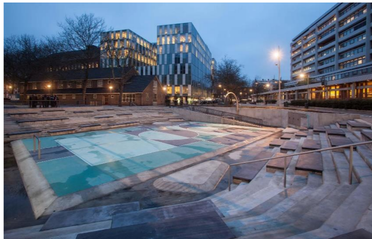
Figure 16: Water plaza used as playing court during dry periods in Rotterdam, The Netherlands (Bravo,
