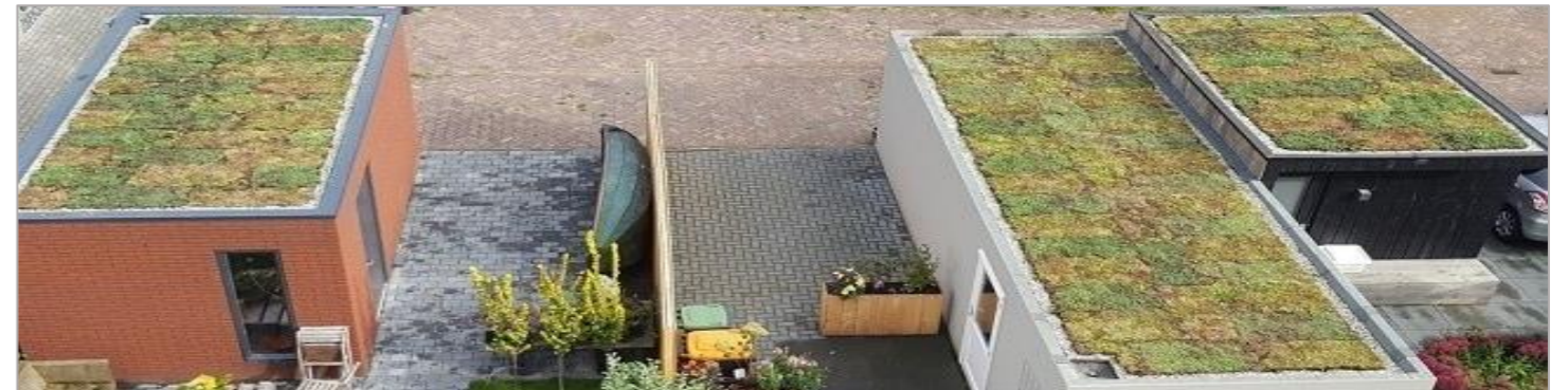
Figure 11: Green roofs at the Havenkwartier neighborhood in Deventer (Deventer stroomt, 2020)
